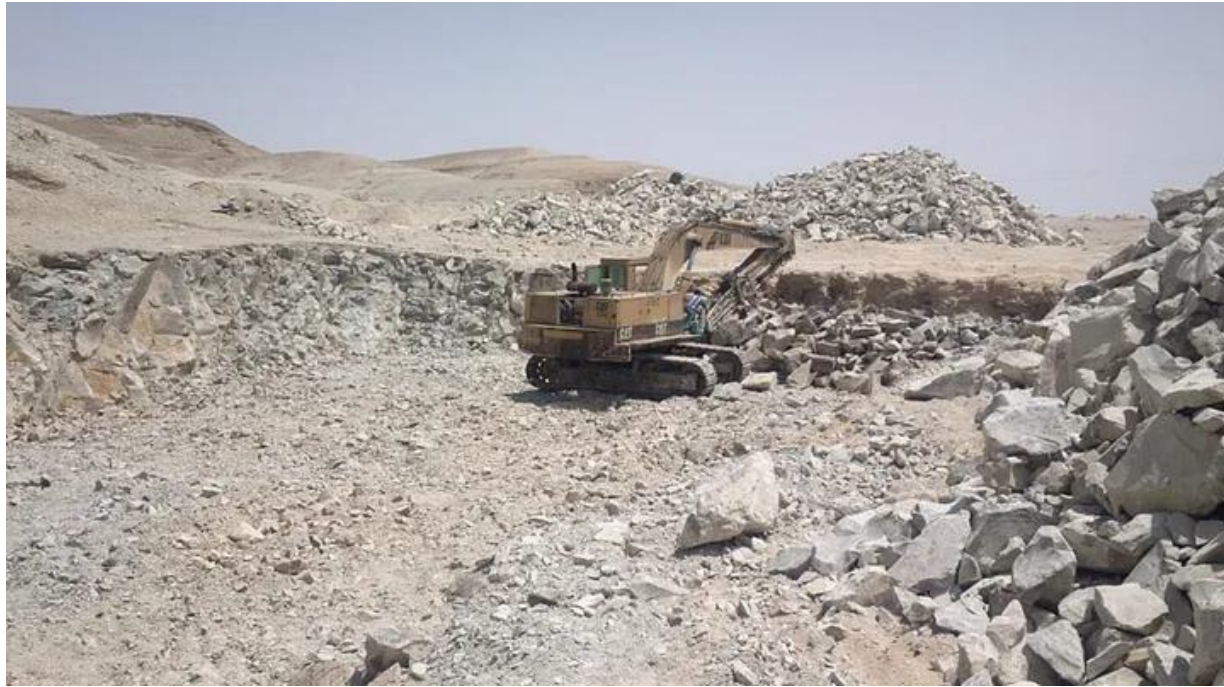
Excavation works at Romana Water Reservoir in North Sinai, Egypt. Photo credit: Chemonics Egypt
