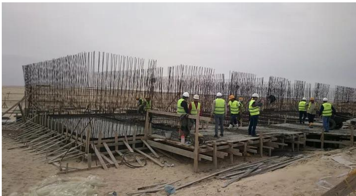
A water desalination plant under construction in Abou El Gouloud, Egypt. Photo credit: Chemonics Egypt
