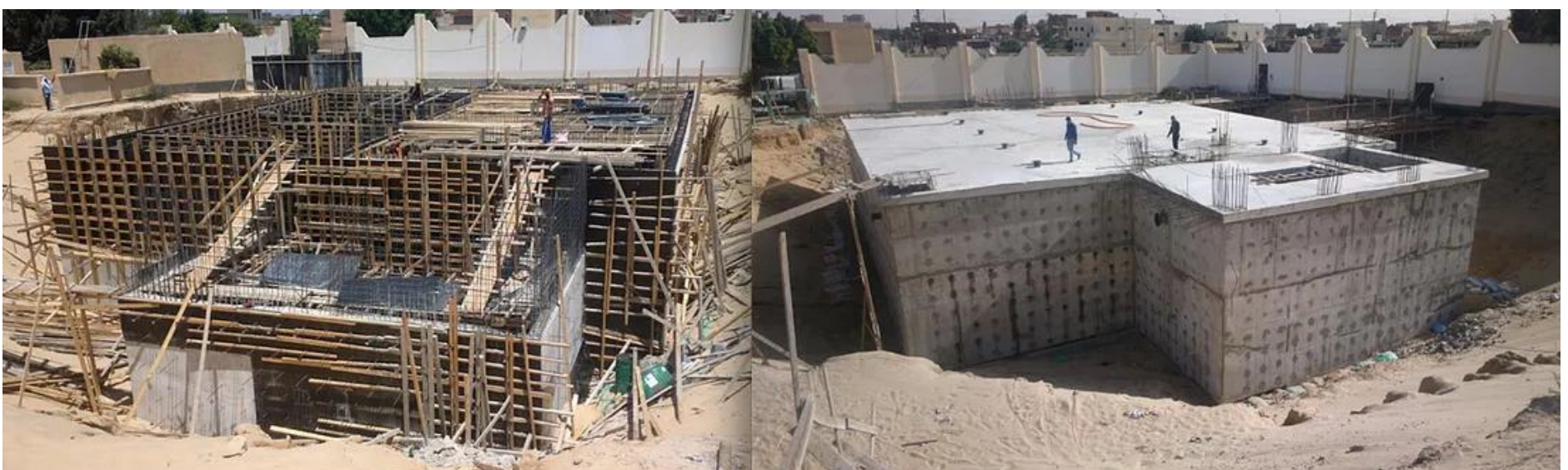
In Beir El Abd, Egypt, a water reservoir under construction (left) and, later, nearing completion (right). Photo credit: Chemonics Egypt
